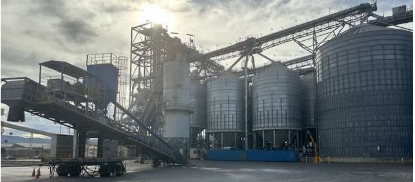
Qube's grain storage facilities, Port Kembla. Source: Auscap
